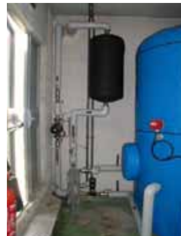
Fig. 10 : Solar collector field for the collective dwelling building in Pessac and drainback tank for the Hotel in Bourges
