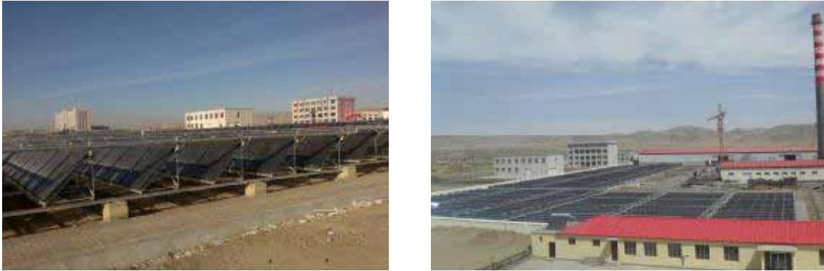
Fig. 6: Solar collector system in solar heating combisystem with seasonal heat storage of Urad Zhongqi
