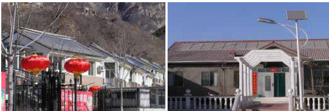
Fig. 7: Solar collector systems on the roofs of peasant houses in Pinggu District of Beijing
