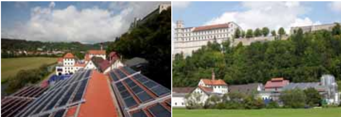
Fig. 3: View on the collector arrays (left) and the storage tanks (right) in July 2009
