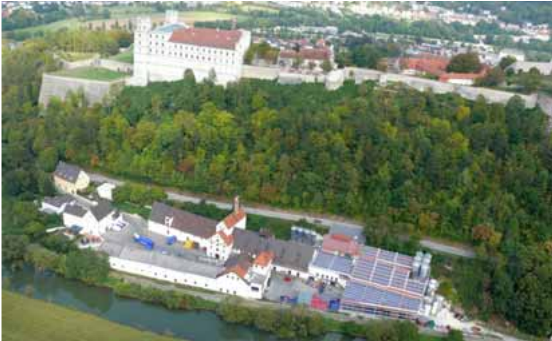
Fig. 2: View on Hofmühl Brewery with the collector arrays
