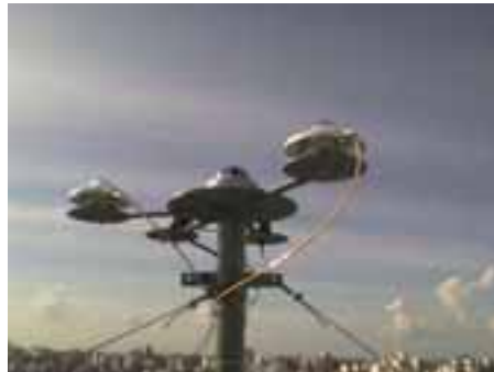
Fig. 5: Measurement tower at FIng (Montevideo).
