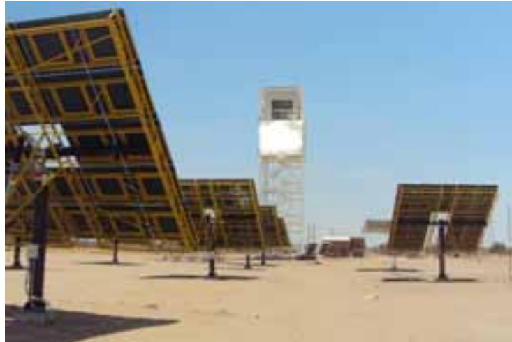
Fig. 2. Picture of the HTF, showing a few heliostats, with the tower, and the laboratory at its base.
