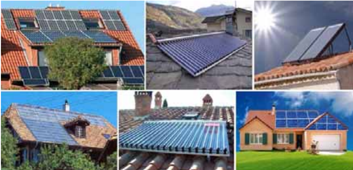
Fig. 1: Current Photovoltaic and solar thermal systems integrations on building roofs.
