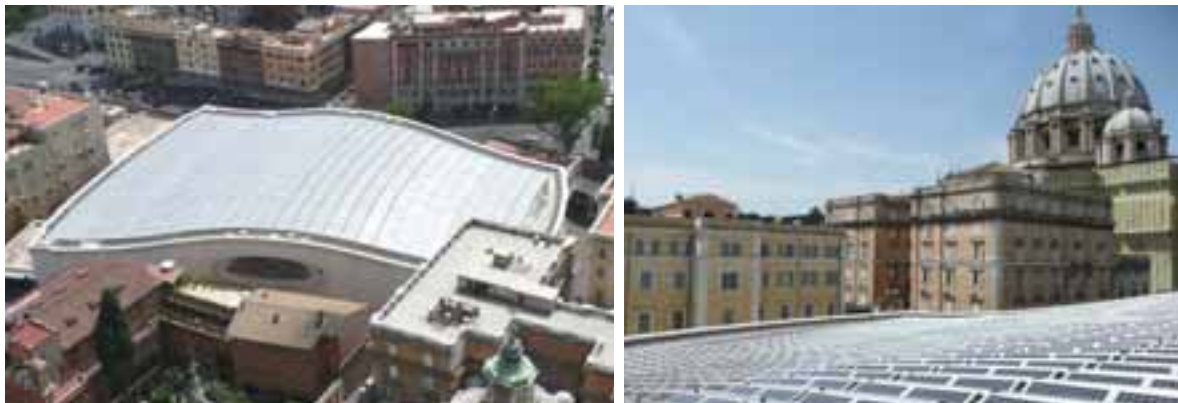
Fig.17 a-b: Exemplary architectural integration of a wide photovoltaic system on an extremely sensitive urban context: Vatican, the Pier Luigi Nervi's Aula.
