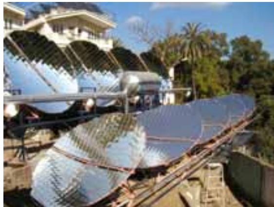
Figure 1: Scheffler Reflector steam system at a Mount Abu hospital in Rajasthan, India.[Source: Heike Hoedt]
