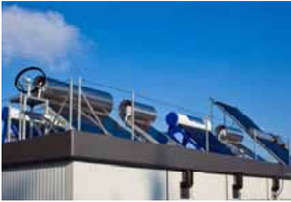
Fig. 6: Roof of the system facility at TestLab Solar Thermal
