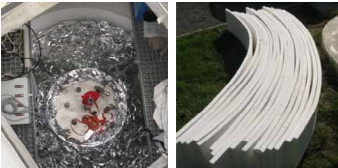
Fig. 2.3: Deconstruction of the first prototype, on the left side storage with compound foil, floating flange and replaced cap insulation – on the right side removed insulation panels of the storage wall insulation
