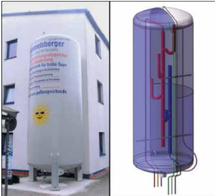
Figure 8: Layout of the real-size storage tank prototype ( 16.4 \text{ m}^3 storage volume) with VSI-insulation: Photograph of the tank (left), sketch of the inner container with supply pipelines and stratification device (right).
