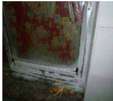
(b) Freezing window pane
