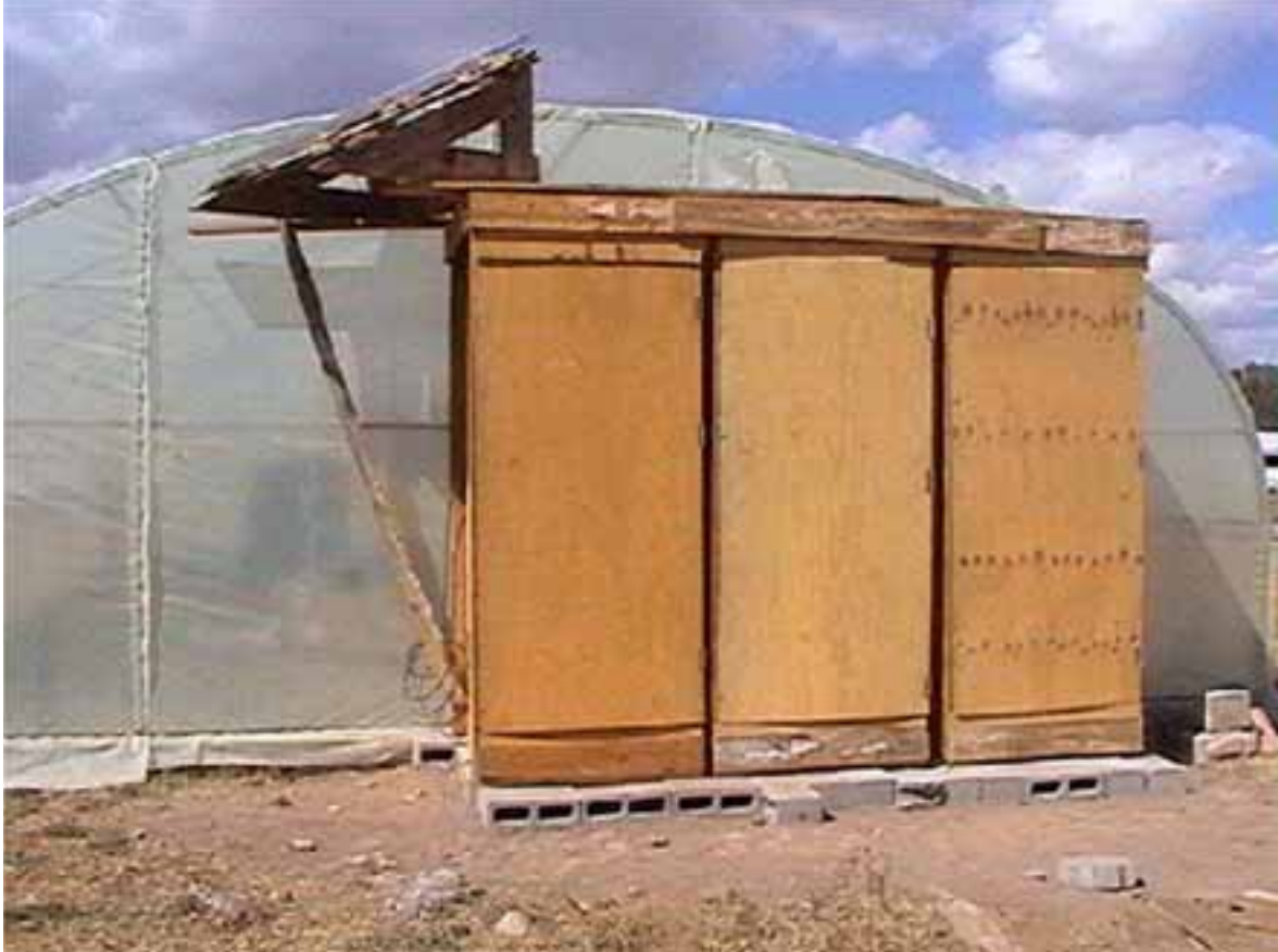
Fig. 5. Solar drier attached to the close end of a greenhouse. It shows the three drying chambers and photovoltaic cells.
