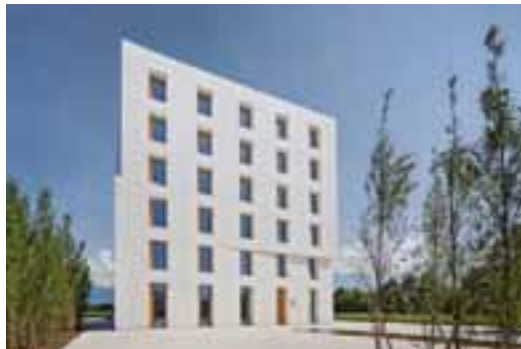
Fig. 1: The realized office building Concept 2226 (Photo: E. Hueber)
