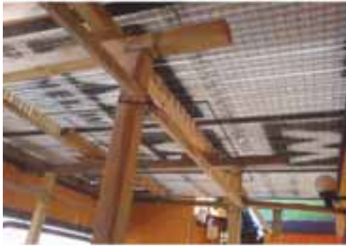
Cover construction process
