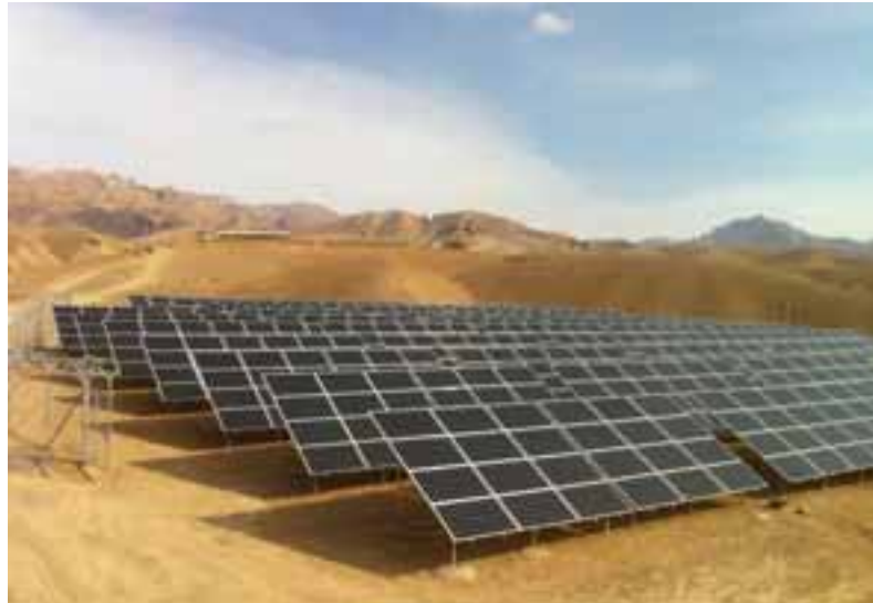
Fig. 2: One of the Large BREP PV Arrays: 300 kWp at the Mullahghulam site
