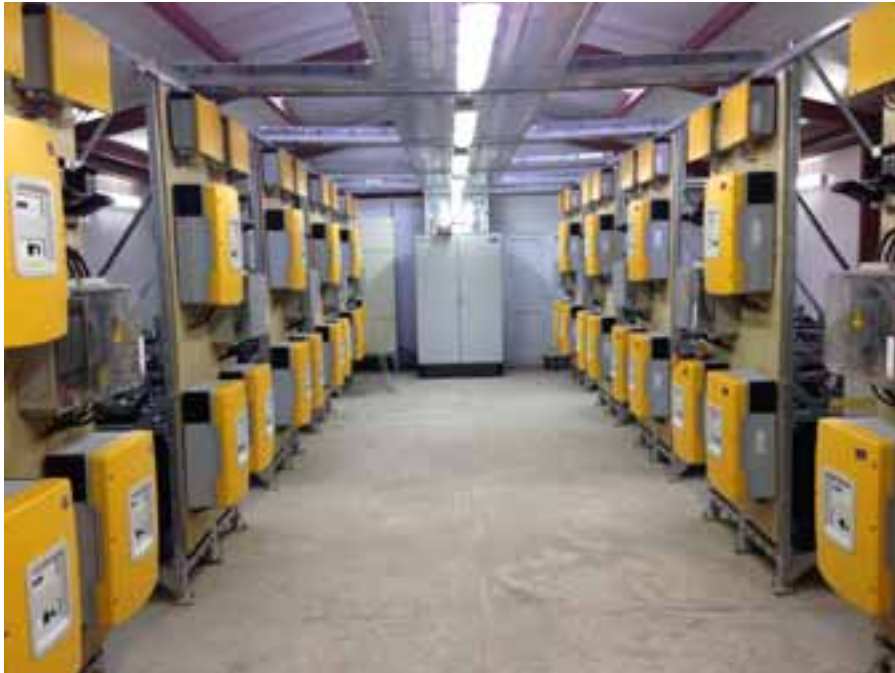
Fig. 5: SMA Multi-cluster Hyderabad BREP Power House with Sunny Island Battery Charging Inverters
