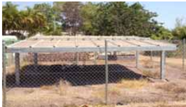
Fig. 1: The Outdoor Solar Facility for the 1.5 kWp CIGS system (ENER TSG200-GS2, Inverter: EnaSolar1.5KWGT-AUNZ) [14]
