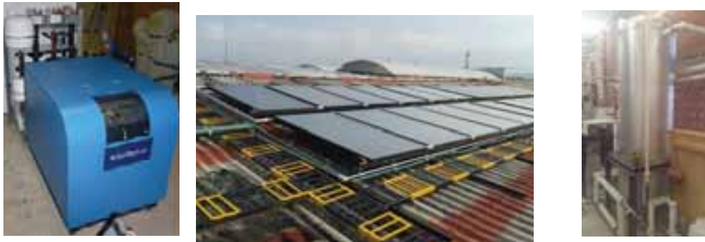
Figure 4. Installing components of solar cooling system
