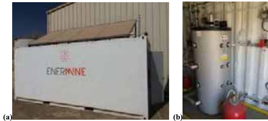
Fig. 2: Pictures of the solar thermal collectors (a) and the storage tank (b) of the pilot plant.
