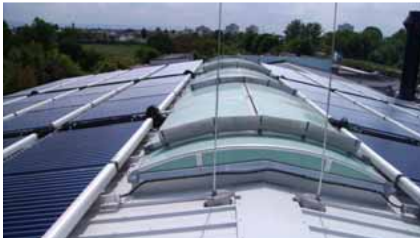
Figure 5: CPC-collector field on metal treatment factory (Holsmöller 2015)
