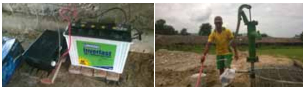
Figs. 15 & 16: PVWP system using a battery and inverter used at a Madi, Chitwan poultry farm in Nepal.
