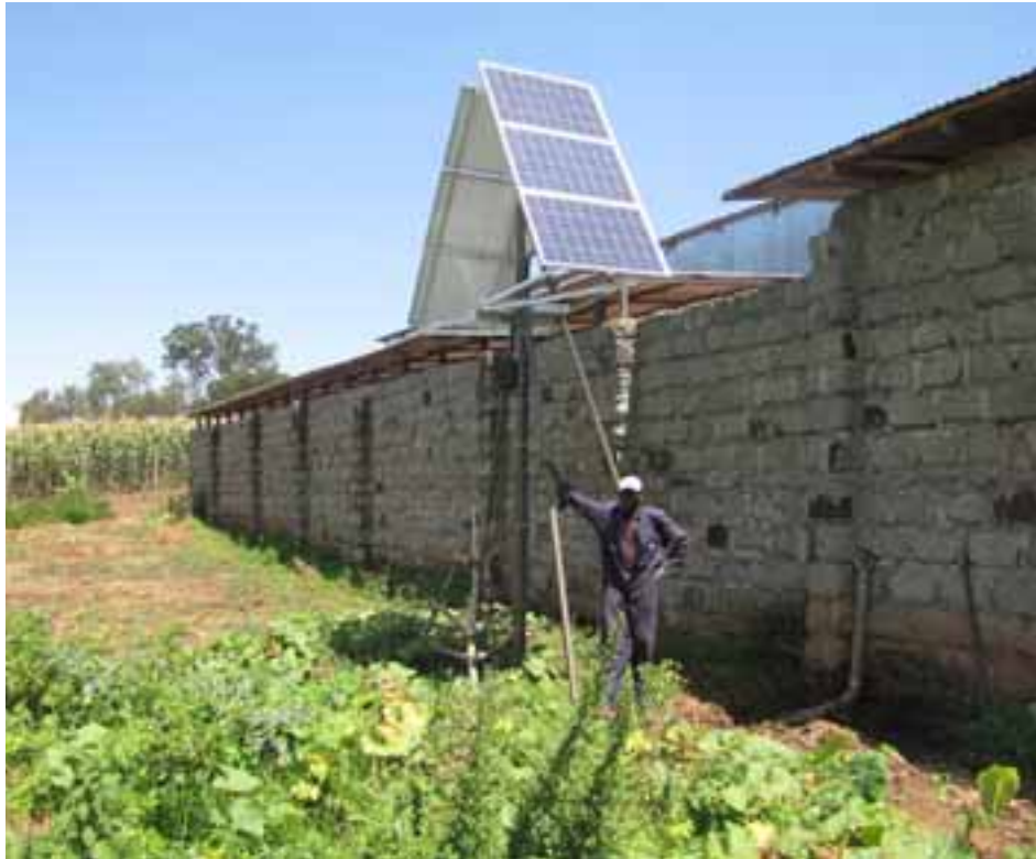
Fig. 5: Dairy farmer from Ngorika shown with his E-W fixed tracking array for a Solar FMC.
