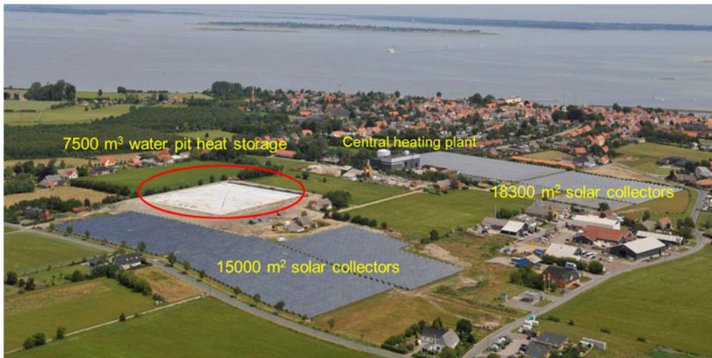
Fig. 1: Bird view of the Marstal Solar heating plant
