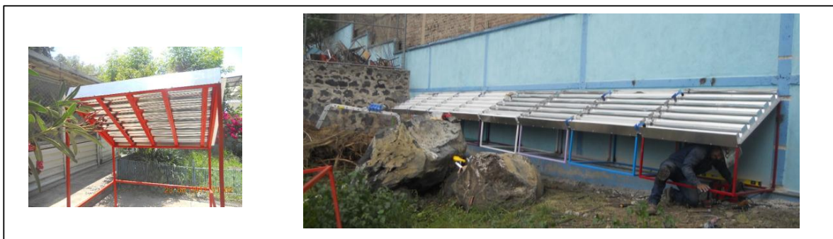
Fig. 11: Parts joint and aliening-fastening on the wall
