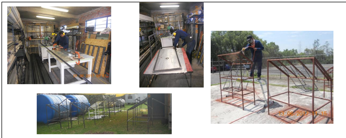
Fig. 8: Metallic structures constructing.
