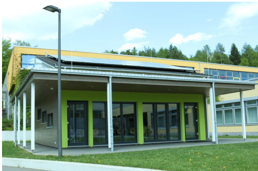
Fig. 1: Front view of the school building
