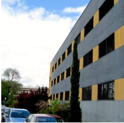
Fig. 2: Administrative offices in Caceres
