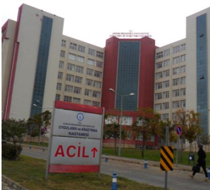
Fig. 4: AHU Hospital in Aydin
