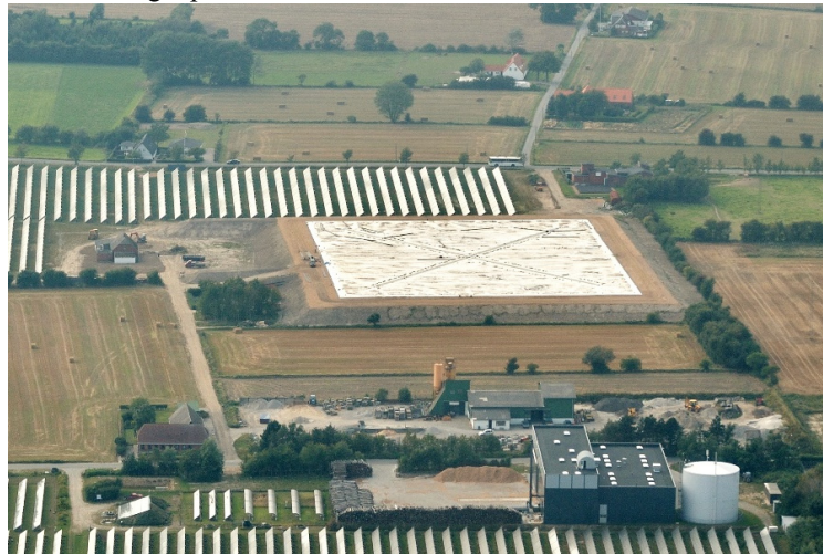
Fig. 1: Bird view of the water pit heat storage in Marstal Solar heating plant
