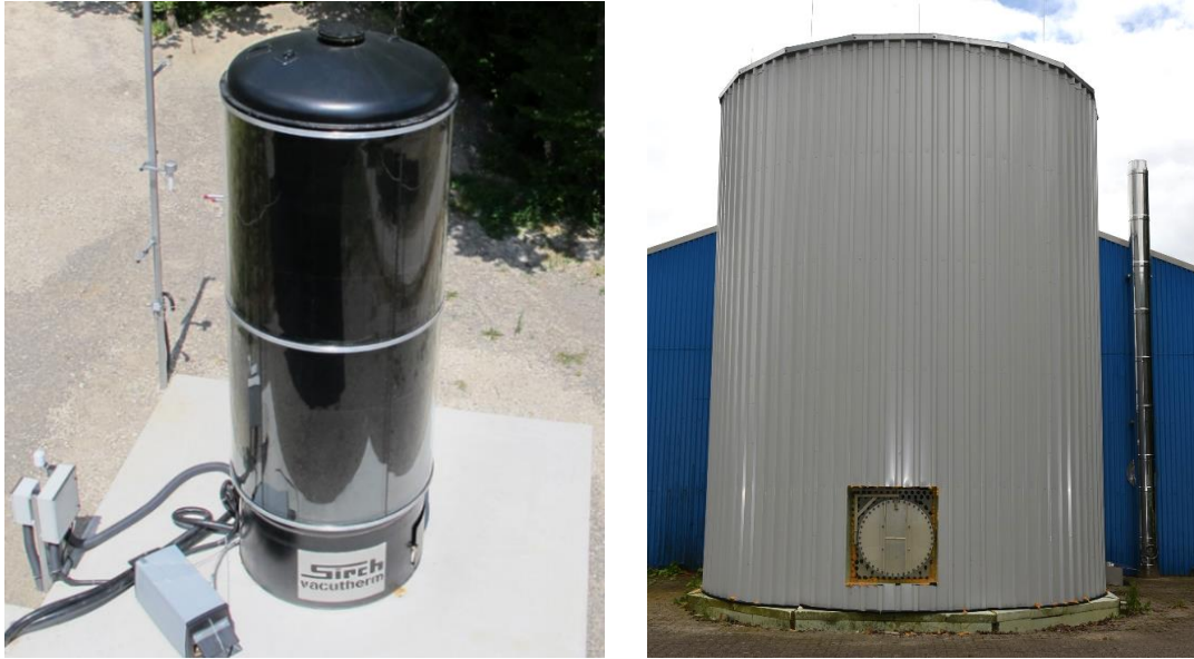
Fig. 1: Outdoor installed thermal energy stores with a water volume of 12 m 3 (left) and 100 m 3 (right)
