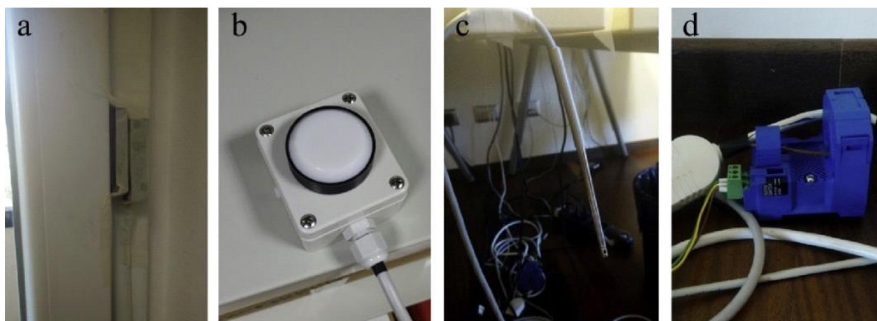
Fig. 2. Sensors installed in each office: (a) opening and closing windows, (b) luxmeter, (c) air temperature probe, (d) ammeter (Pisello et al., 2016).
