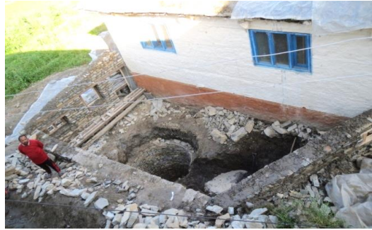
Fig. 8: Heating water for increased anaerobic process in the production of biogas and heating a high-altitude greenhouse.
