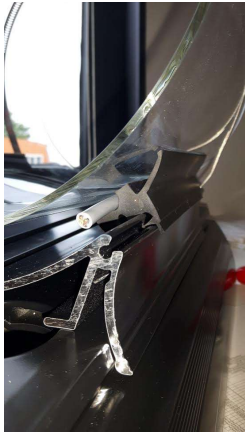
Fig 9. Detail of the tube on the aluminium profile
