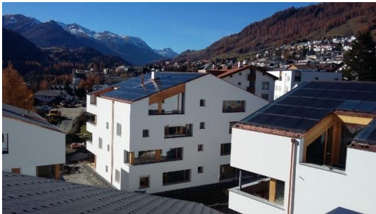
Figure 9: P&D project Sotchà in Scuol (CH). Roof-integrated PVT plant for the regeneration of boreholes (Vassella & Baggenstos, 2015).
