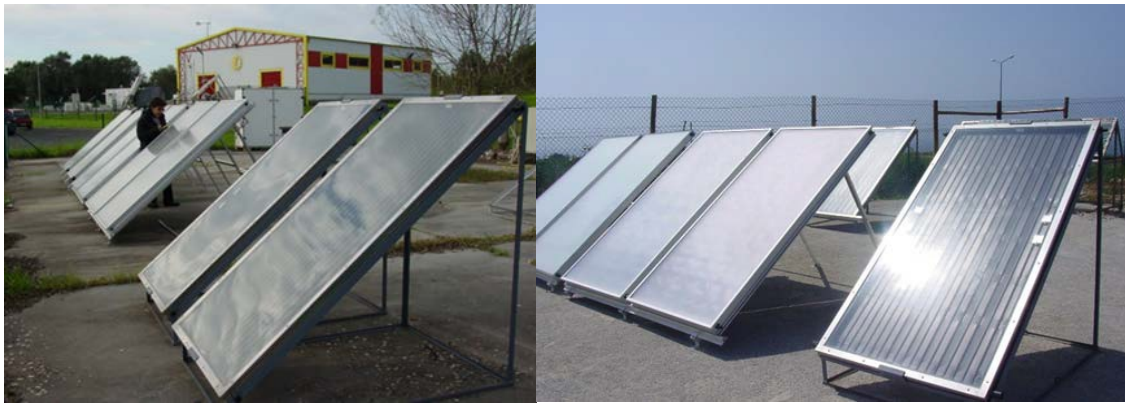
Fig. 1: Installation of collectors in OET sites - Urban (left); Maritime/Industrial (right)
