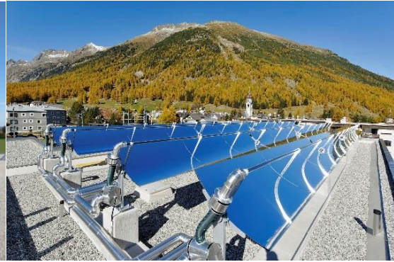
Fig. 2: SPHP in Bever, 1700 m above sea level, 115 m 2 (aperture) PTC-collectors, axis orientation NS with 19° deviation clockwise
