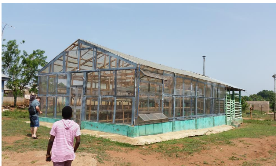
Fig. 1. 5tonne capacity dryer located in Ejura
