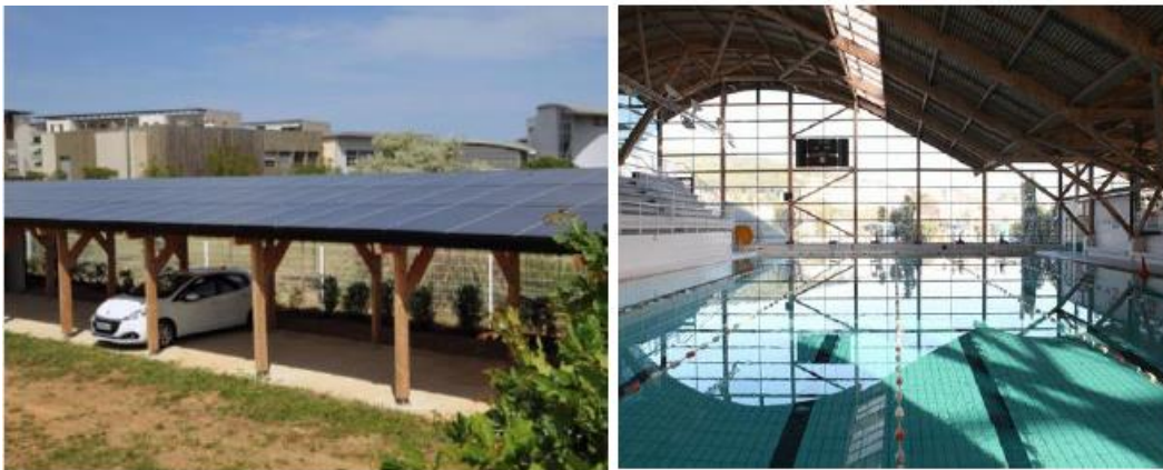
Fig. 2: picture of the PV/T canopy for the municipal swimming pool of Sète (France)
