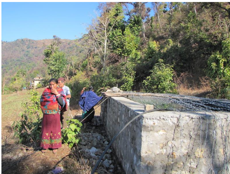
Fig. 11: Pokharikada main water storage tank for solar water pumping from a spring for irrigation.
