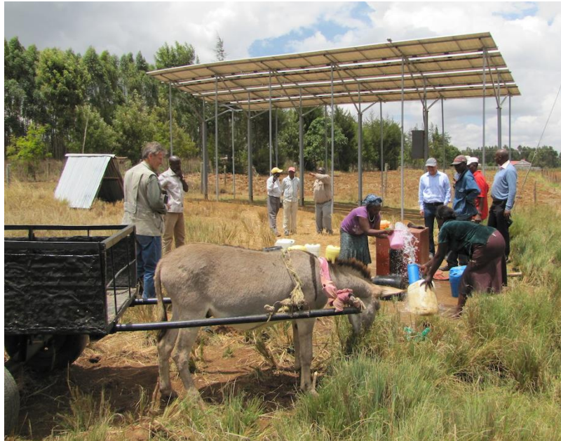
Fig. 6: Lorentz helical rotor 8.1 kW p solar water pumping system providing community and irrigation water supply to 500 farmers in Nyandarua County. The borehole is 230 meters.
