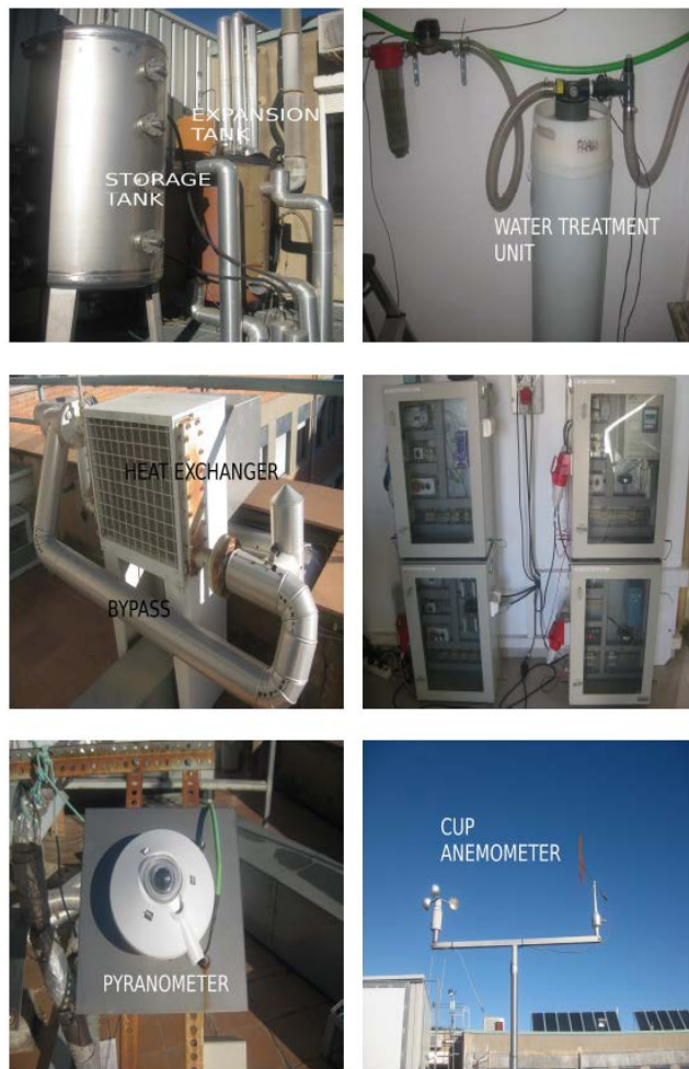
Fig. 6 Pictures of the key elements constituting the CTTC Solar Cell.
