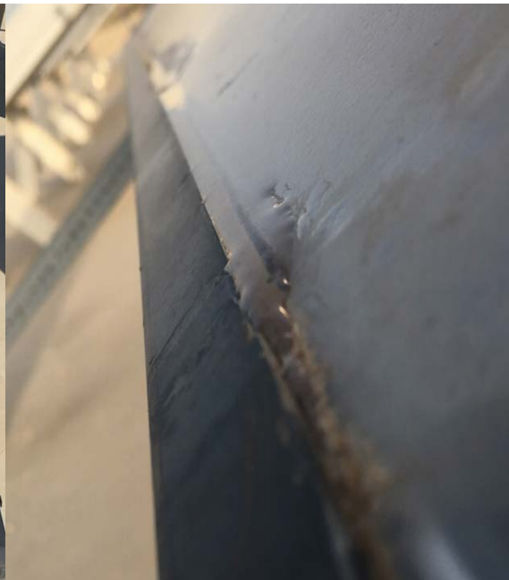
Fig.6: When dew flows down the glass surface it will reach the lower edge of the frame. Dust that has been picked up by the dew will accumulate there.
