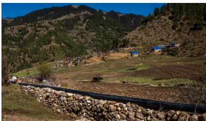
Fig. 4: Elevated Section of Penstock
