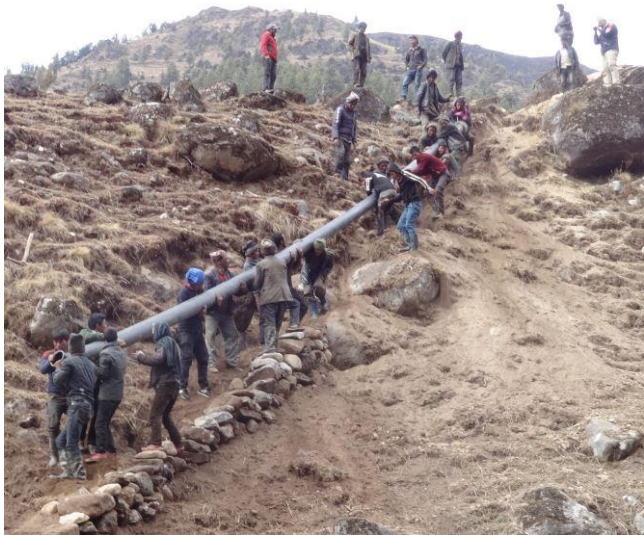
Fig. 15: Laying Penstock in Steep Section
