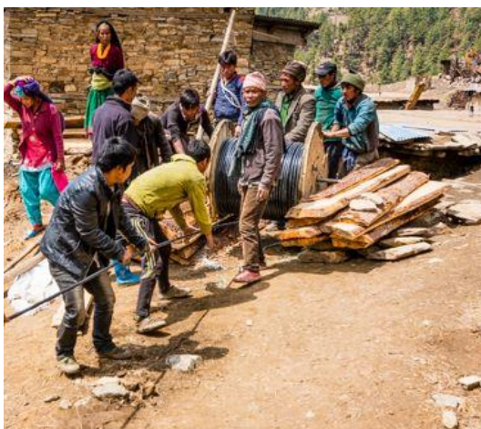
Fig 7: Unwinding Armored Transmission Cable from the Spool
