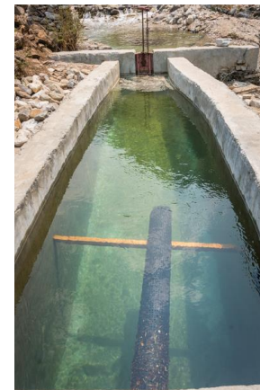
Fig. 2: Three Dimensionally Shaped Settling Pond
