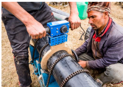
Fig. 3: Thermally Welding the Penstock
