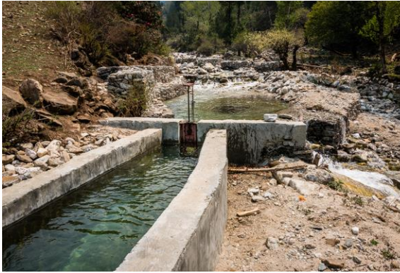
Fig 1: Two Levels of Sedimentation Tanks
