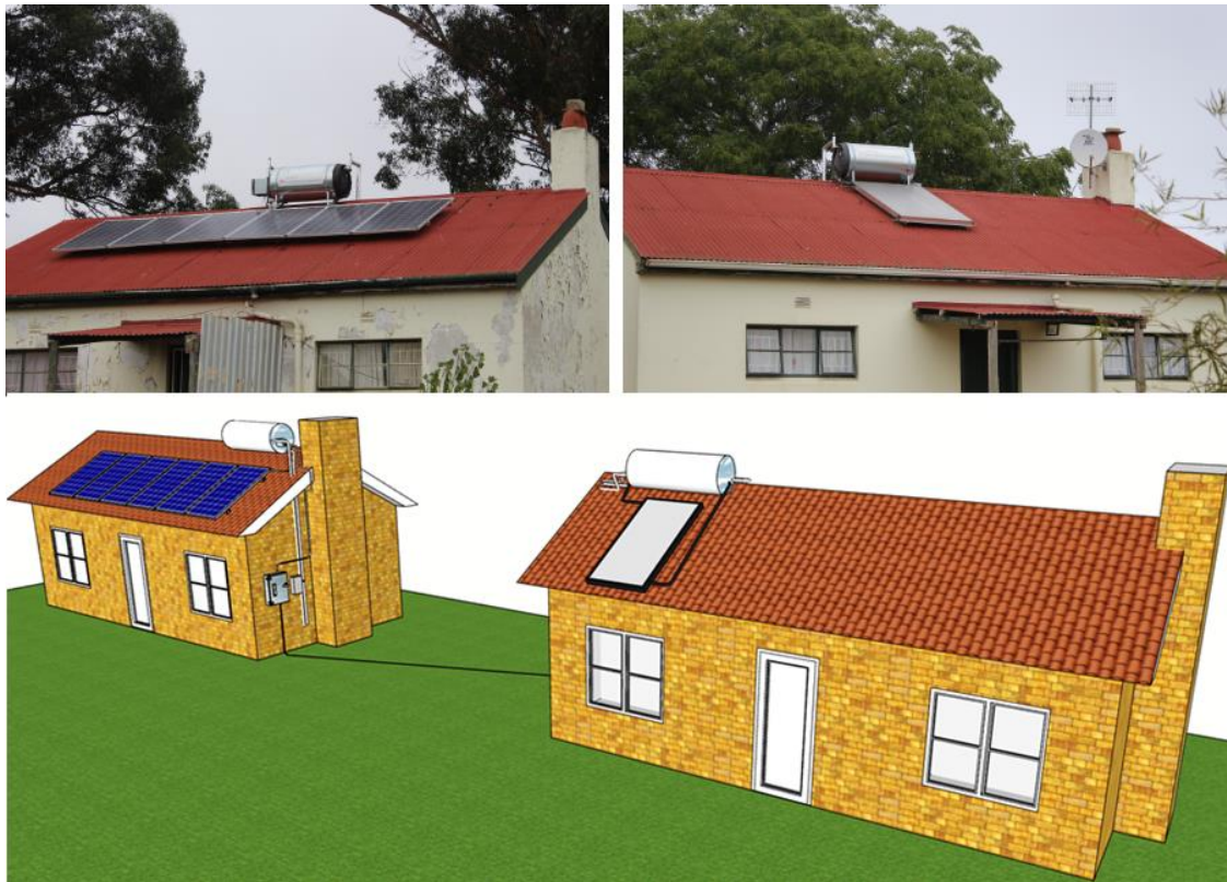
Figure 1: PV hot water and SWH system installed at Mariendahl Farm residence in Western Cape, South Africa (SketchUp Free)
