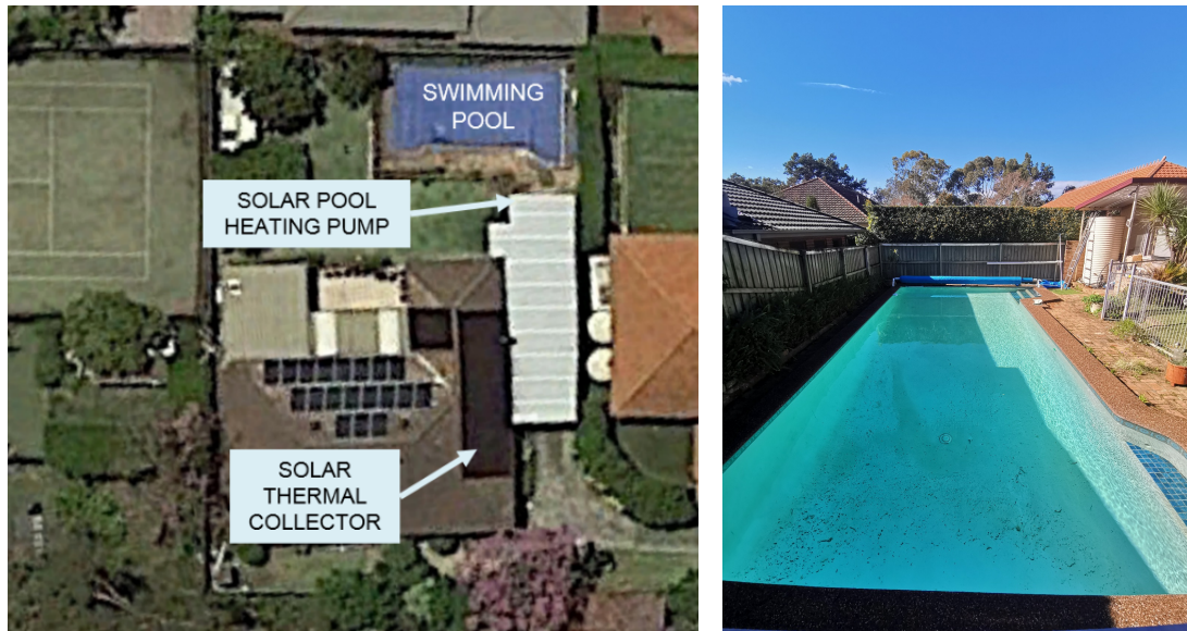
Fig. 1 Overview of the residential solar pool heating system.
