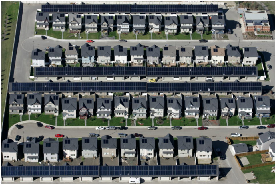
Fig. 3: Aerial view of Drake Landing Solar Community
