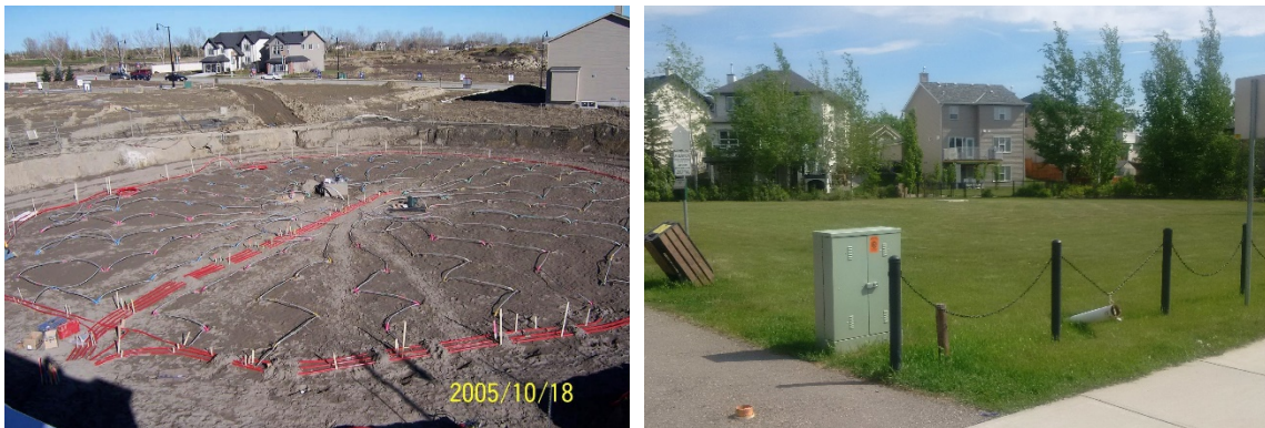
Fig. 4: Borehole field under construction and currently, as a landscaped park
