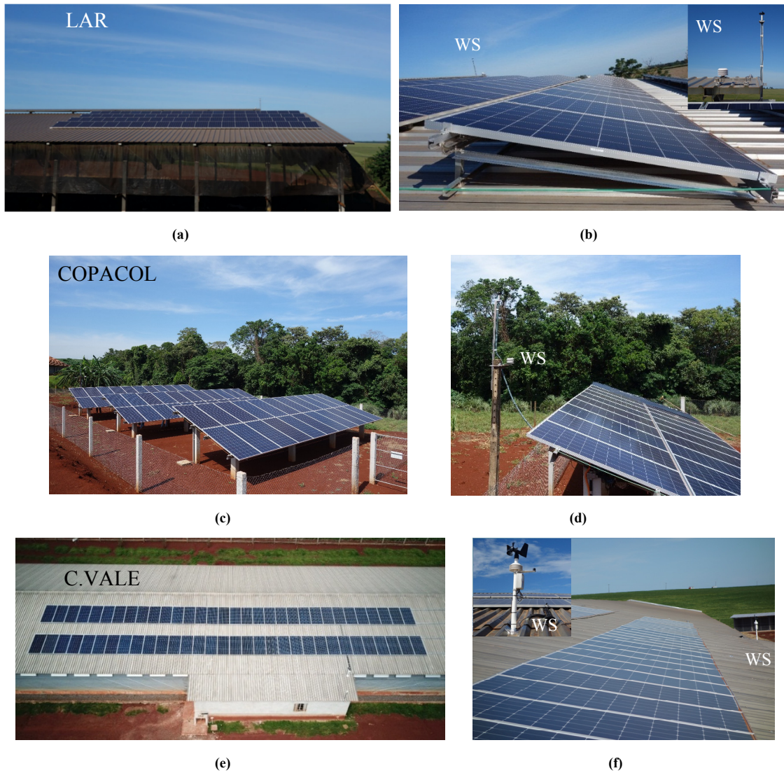
Fig. 1: The 20 kWp PV systems installed and analysed: (a) dairy farm, PV array on a north-facing sloping roof, 18° tilted (8° above to the roof slope), azimuth of 8° NE (Medianeira-LAR); (b) detail of the PV module installation and weather station (WS), LAR; (c) PV system installed in a poultry farm, ground mounted PV, 18° tilted, north-oriented (Cafelândia-COPACOL); (d) detail of the position of weather station, COPACOL; (d) PV system installed in a poultry farm, PV array mounted on the rooftop, 13° tilted, azimuth of 52° NE (Assis Chateaubriand – C.VALE) and (f) details of the PV module installation and weather station, C.VALE.
