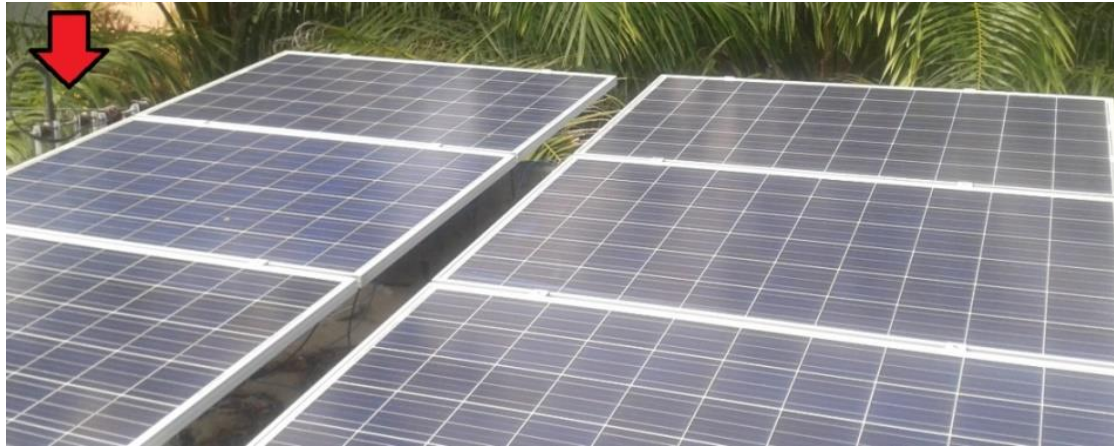
Figure 2: PV DG installed in the LEA / UFC and the network connection point of the Pici Campus.
