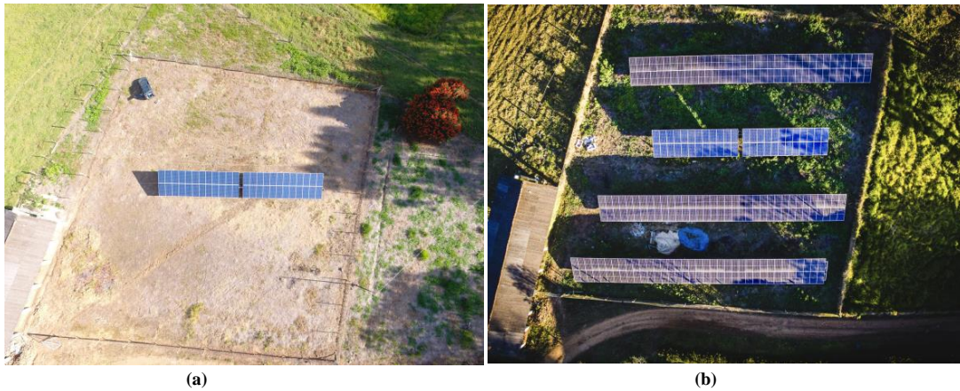
Fig. 3: (a) Enercred first power plant (15 kWp) and (b) Enercred PV system expansion (75 kWp)
