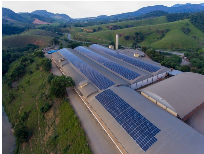
Fig. 9: Sicoob Credit System from ES 1 MWp PV system to be connected to the grid by the end of 2019.
