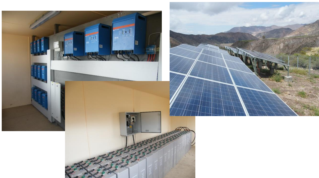
Fig. 2: Principal components of 34 kWp PV off-grid system (Putre, northern Chile)
