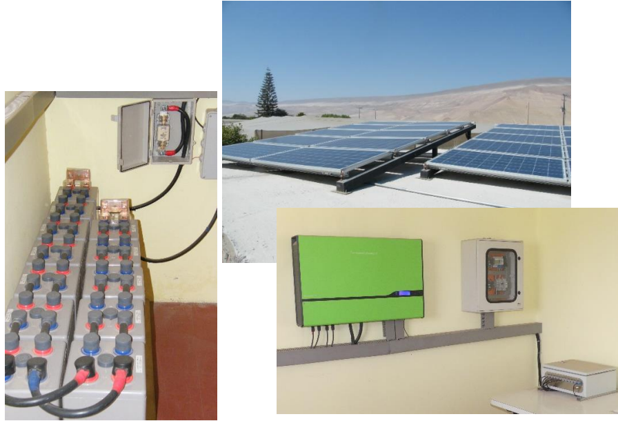
Fig. 8: Principal components of 5 kWp PV on-grid system with storage (Azapa, Arica and Parinacota Region)
