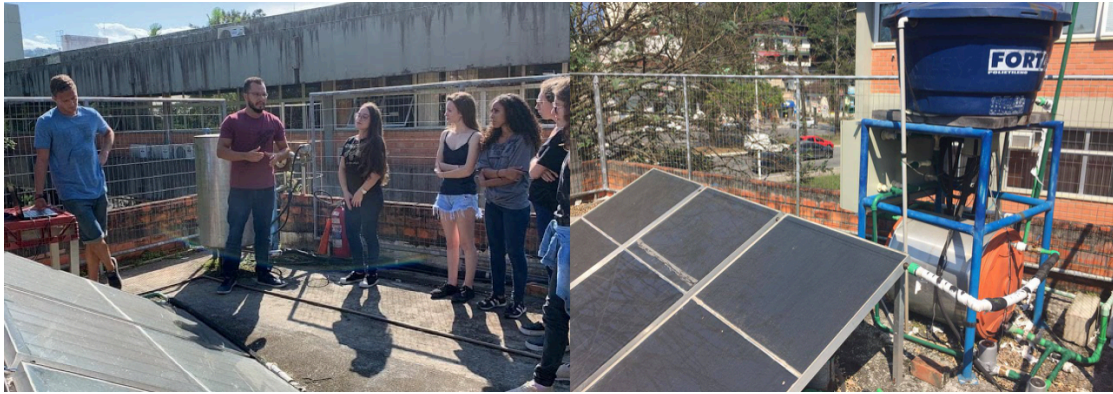
Fig. 3: GPER Solar Plant Lab.
