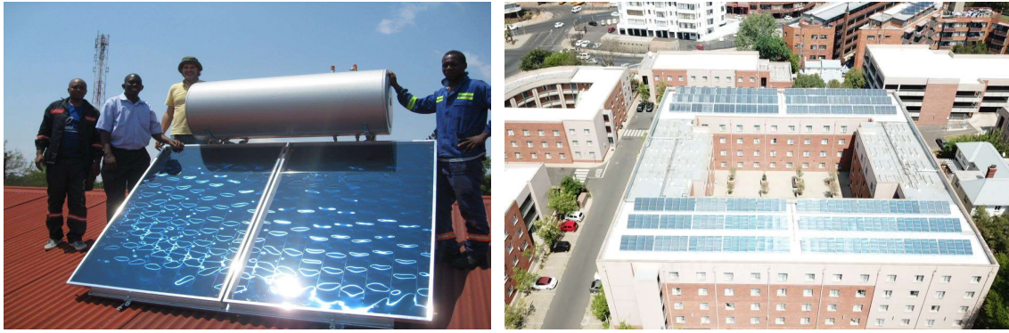
Fig. 4: The size of the demonstration plants installed in the course of the project ranges from 2m 2 to 600m 2 collector area
