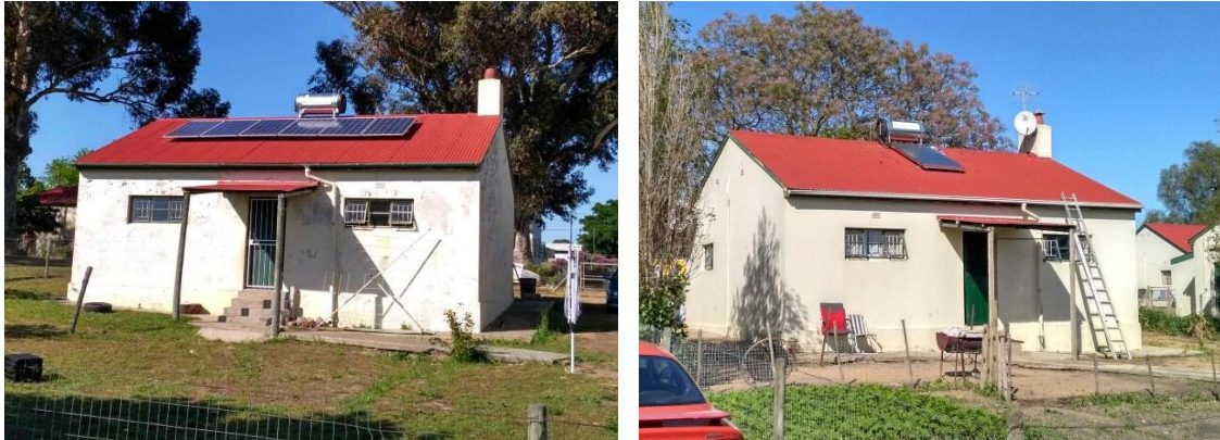
Fig. 6: Direct PV-supplied hot water system (left) and conventional thermosiphon system (right) in an experimental set up
