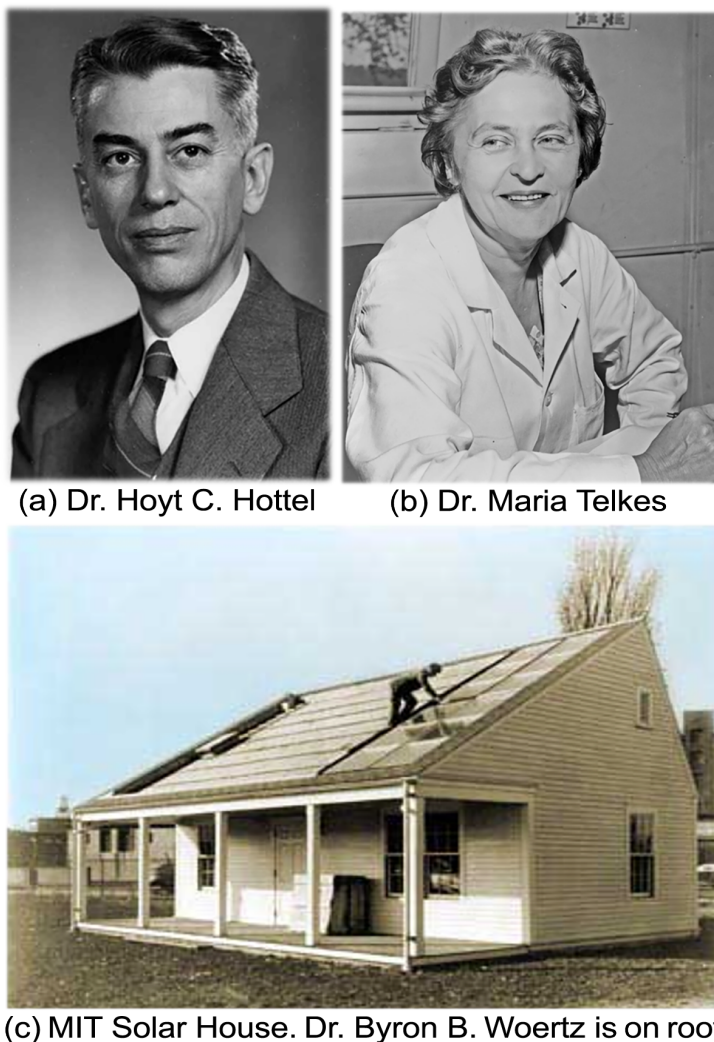
Fig. 3: Early pioneers: (a) Dr. Hoyt C. Hottel (1903-1993); (b) Dr. Maria Telkes (1900-1995), co-designer of MIT house; (c) MIT 1 st Solar House (1939)-first “soiling laboratory,” with Dr. B.B. Woertz working on heat collector on the roof.
